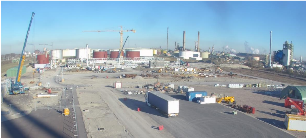
Picture 1 : Aliphos Dunkerque Site under construction
