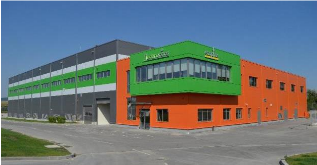
Picture 3 : Technophos building in Devnya (Bulgaria)
